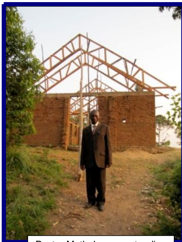
Pastor Muthahanzwa standing outside the almost completed building at Kikyo Baptist.
